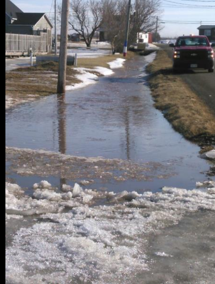
Inondation rue Niles Street flooding
