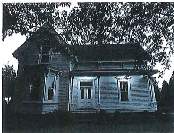
Fig C: House at 89 Route 133
