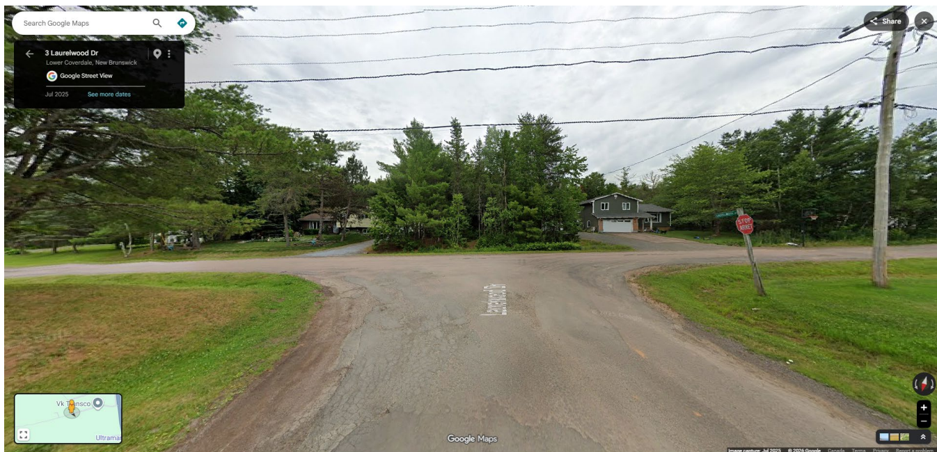
View of the unbuilt section of Laurelwood Drive. / Vue de la portion non-construite de la promenade Laurelwood.
