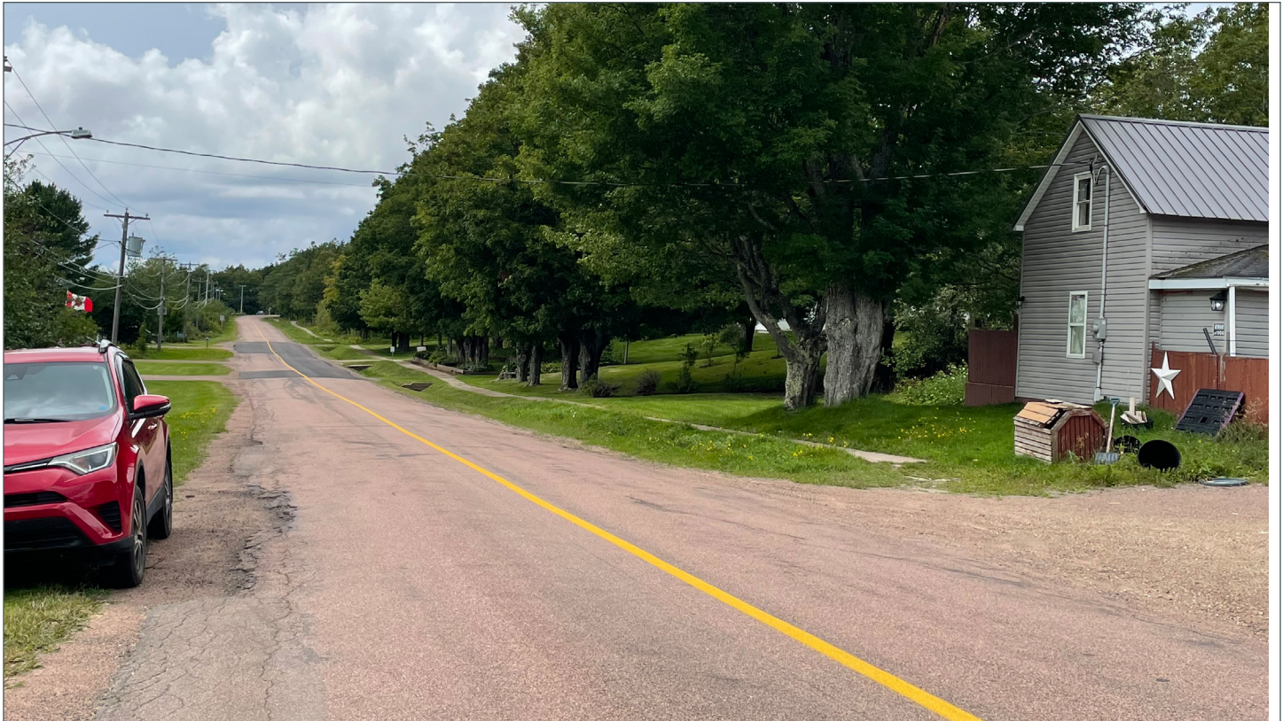
Woodlawn Road, looking southwest
