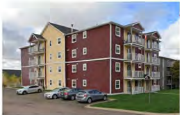
Existing four-storey apartment building.
